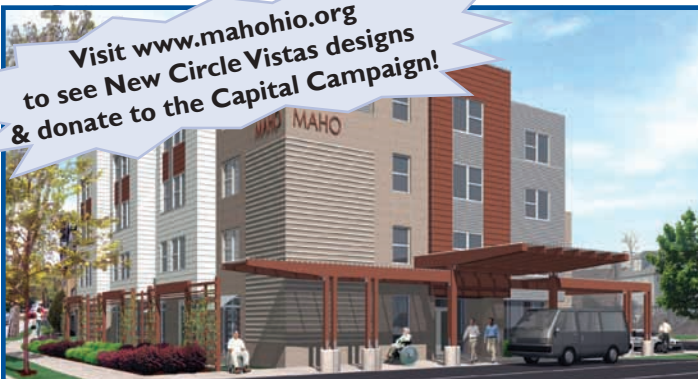
The main entrance of New Circle Vistas.
